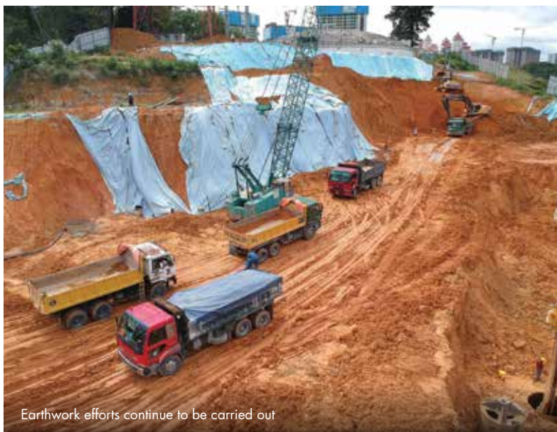
Overview of construction site where The MET will be built
